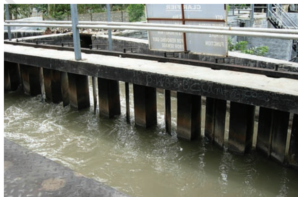
Fig. 18.4 Grit and sand removal tank
