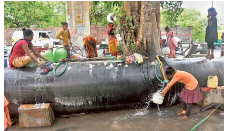
Women filling drinking water from a leaked pipeline of Delhi Jal Board at Ridge Road near Dhaula Kuan on Thursday. •SHIV KUMAR PUSHPAKAR
