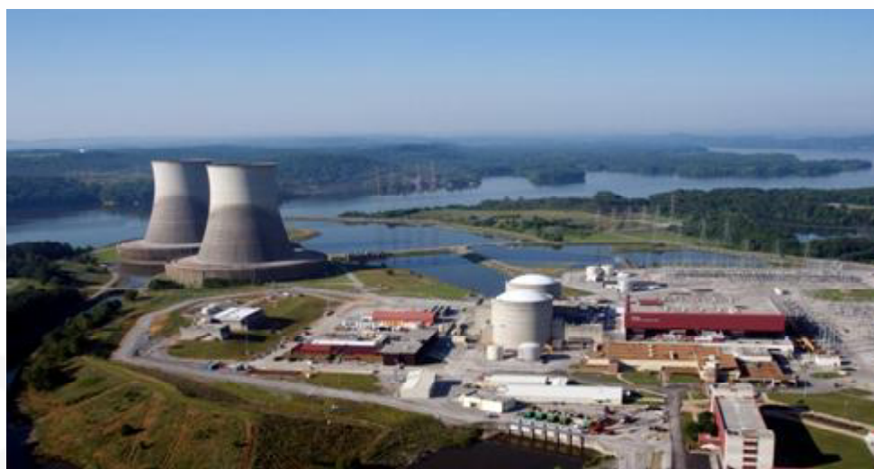
Fig. 7.13: A view of atomic power station.
