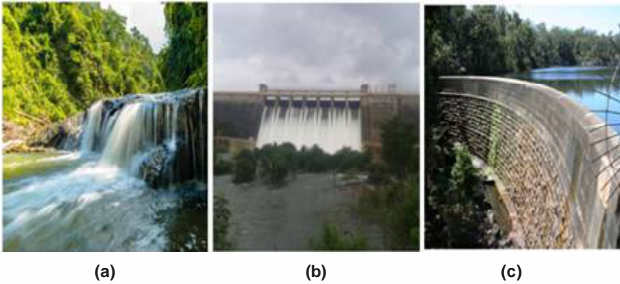
Fig. 4.12: a) Drainage system for preventing uncontrolled flow of water; b) & c) Check dams for preventing the flow of running water.
