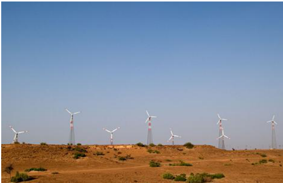
Fig. 7.10: Use of renewable energy as wind pump.
