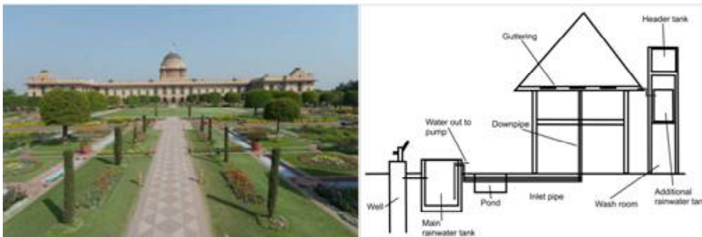
Fig. 4.5: Rainwater harvesting in Rashtrapati Bhawan.
