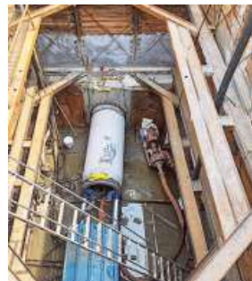
Microtunneling work under way at Anand Vihar RRTS station. • PTI
