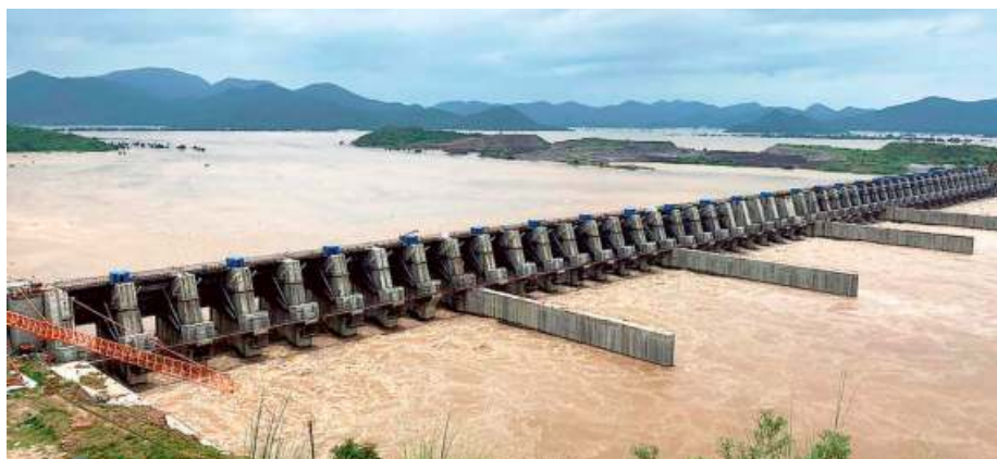
Alert mode: Water gushing through the gates of the Polavaram project in West Godavari district of Andhra Pradesh on Sunday. *SPECIAL ARRANGEMENT
