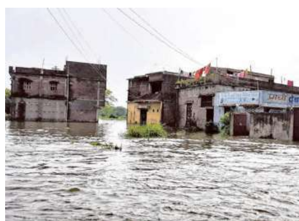
Cause for concern: Buildings surrounded by flood water in East Champaran, Bihar. *SPECIAL ARRANGEMENT
