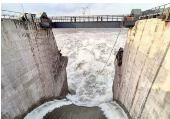
What a rush! Water gushing out after radial gate of KL Rao Sagar Pulichintala Project was washed away. ■ T. VIJAYA KUMAR
