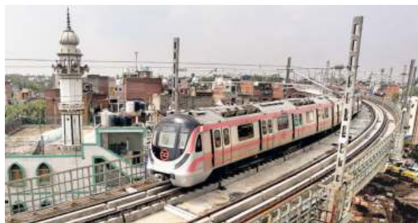
A Metro train passes through Trilokpuri on the Pink Line in the city on Friday. *R.V. MOORTHY
