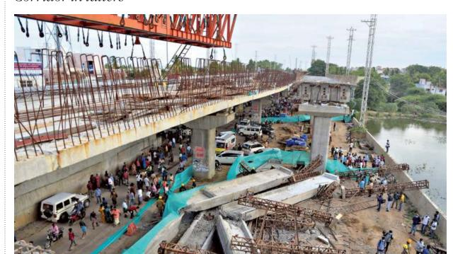
A portion of the under-construction elevated highway came crashing down on New Natham Road in Madurai on Saturday. Officials said one of the cables of a hydraulic jack snapped, leading to the collapse of a 70-tonne girder. A worker hailing
