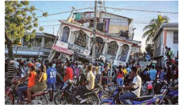
People outside the Petit Pas Hotel, destroyed by the earthquake in Les Cayes, Haiti, on Saturday. • AP
