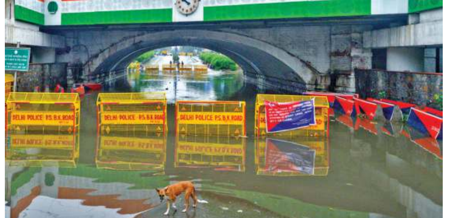
No entry: A waterlogged Minto Bridge remained closed to traffic till noon following heavy rain in New Delhi on Saturday. • R.V. MOORTHY (REPORT ON PAGE 2)
