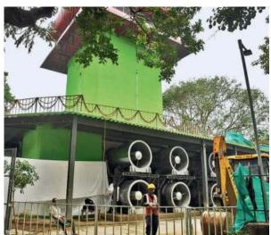
The smog tower has 40 fans and 5,000 filters to clean the air.
