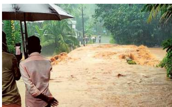
No respite: The flooded Angamoozhy-Kottamonpara bridge in Pathanamthitta on Saturday. ■ LEJU KAMAL
