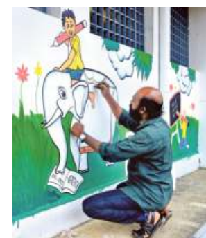
Final touches being given to a primary school in Kottayam on Saturday.
