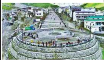
>> Platform constructed at Sangam Ghat
